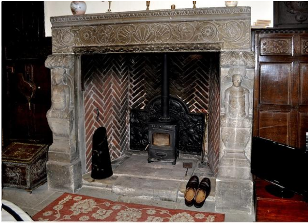
Figure 3 The Tan House fireplace with carved jambs supporting a carved stone lintel.
